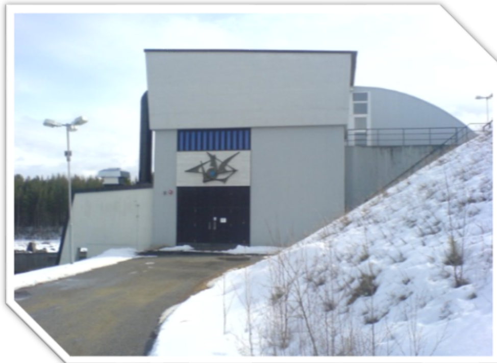
Hermansboda hydro power plant
